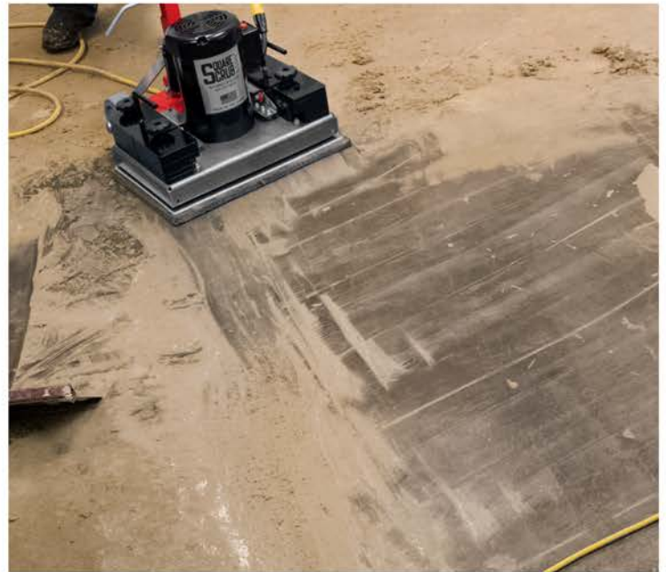
The Square Scrub ® Pivot and the SAP, Square Abrader Plate, can save hours by adding the orbital cleaning power of the Pivot! The Carbide Tungsten tips of the Square Abrader Plate make quick work of linoleum, glue, or paint on floors!
