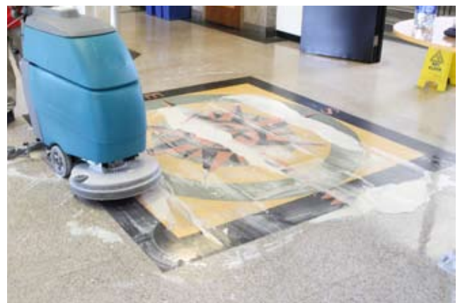
Using an autoscrubber to clean slurry
